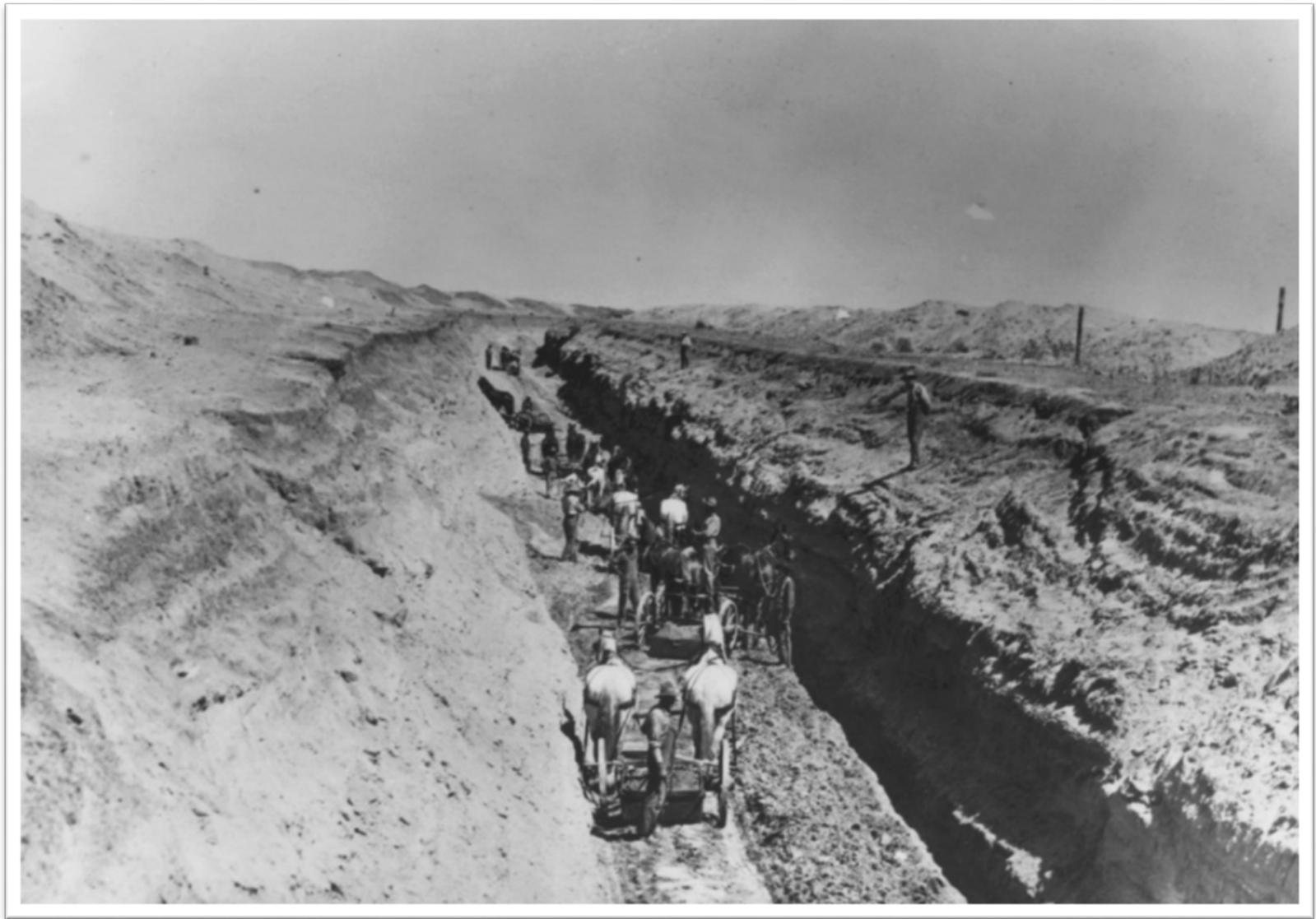
Bijou Irrigation Ditch - Colorado
