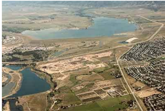
New Reservoir Construction
